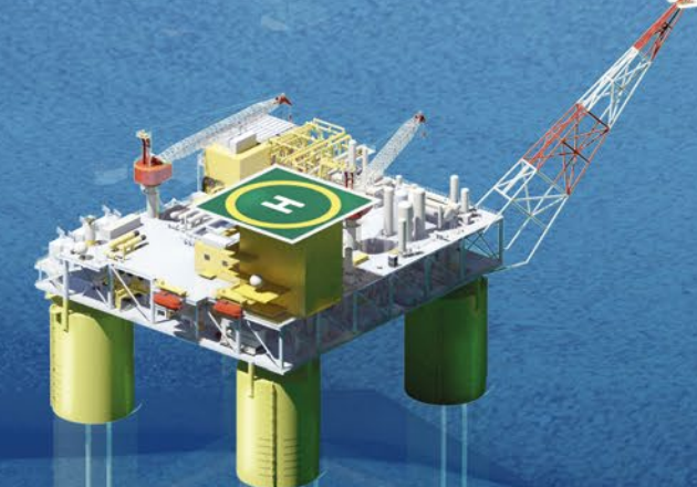
▶ Extended Tension Leg Platform (ETLP)
