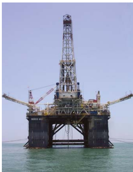
SPC and partners have begun drilling of the Jeruk-3 well
