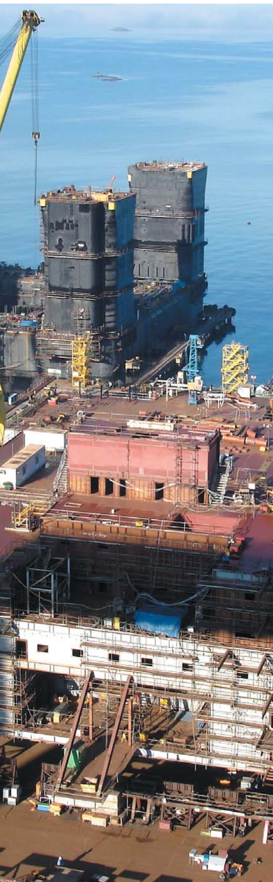
The 13,000-tonne deckbox inches into position above the barge FS-1 (top picture), as P-51 prepares for the marine mating of its topside (bottom picture, front) and lower hull (bottom picture, behind)
