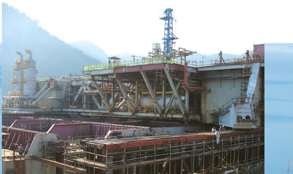
The 13,000-tonne deckbox inches into position above the barge FS-1 (top picture), as P-51 prepares for the marine mating of its topside (bottom picture, front) and lower hull (bottom picture, behind)
