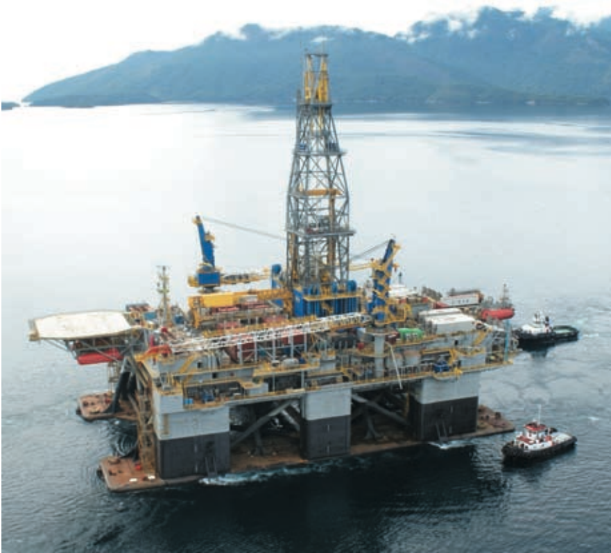
Noble Dave Beard on its way to BrasFELS in March 2009 for completion works
