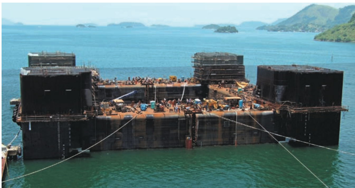
BrasFELS' technological capabilities and technical expertise are key in the successful joining of the two 'C' sections of the lower hull of P-56
