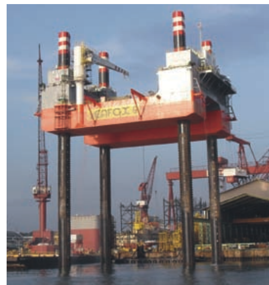
Seafox 6 in mint condition after undergoing conversion works at Keppel FELS
