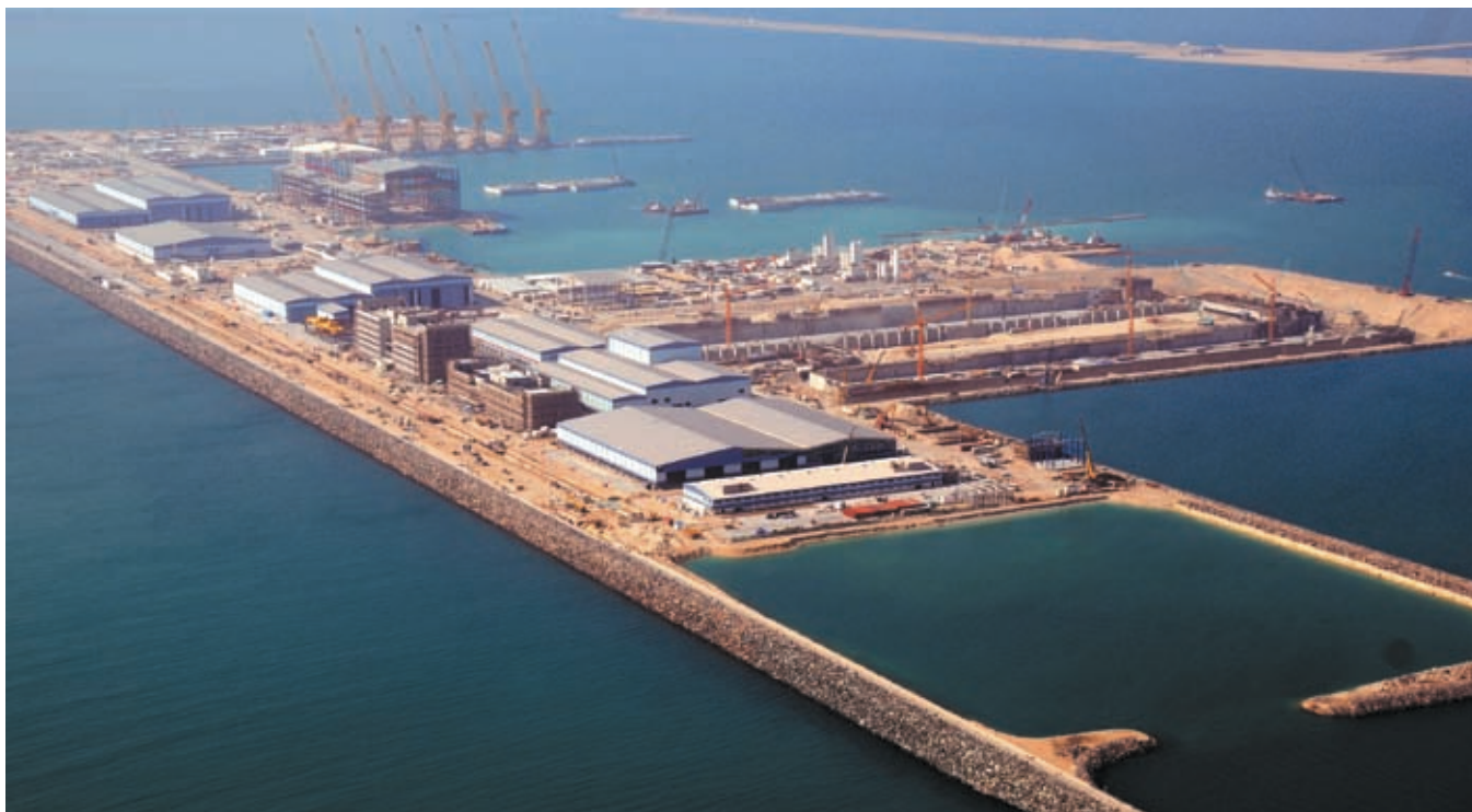
When operational, Nakilat-Keppel O&M will operate in all sectors of the shiprepair industry and will have some 80 drydocking projects a year
