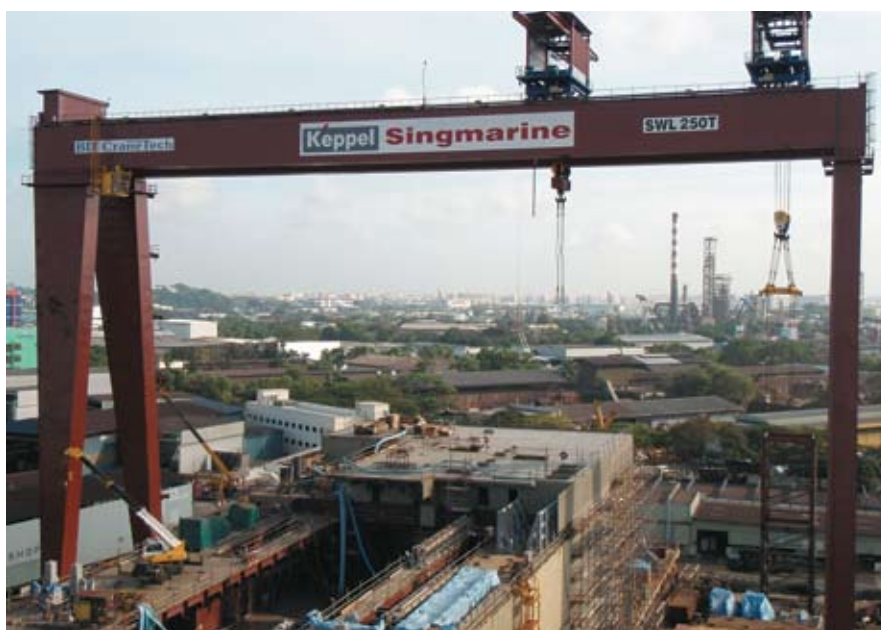
The 250-tonne gantry crane has improved productivity at Keppel Singmarine significantly since it commenced operations in February last year
