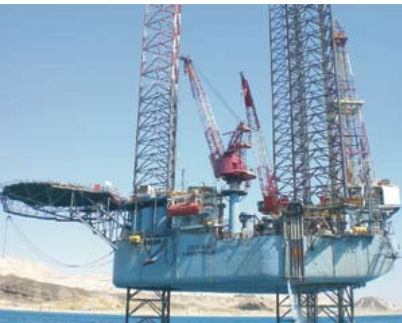
Ocean Heritage returns to operational mode following timely repairs by Keppel FELS's offshore repair specialists, the Flying Squad
